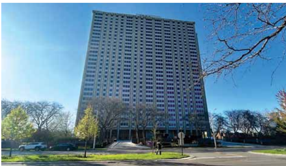
The 1300 Lafayette building is a 1960s-era 30-story co-op housing building in Detroit. | NICK MANES
