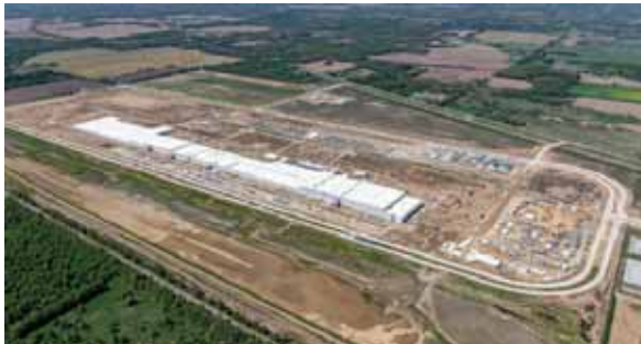
An aerial view of Ford's BlueOval Battery Park in Marshall under construction, taken May 8. (WALBRIDGE VIA FORD MOTOR CO.)
